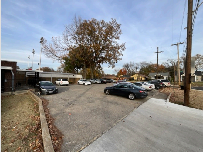
OVERVIEW OF ACCESSIBLE PARKING AREA
