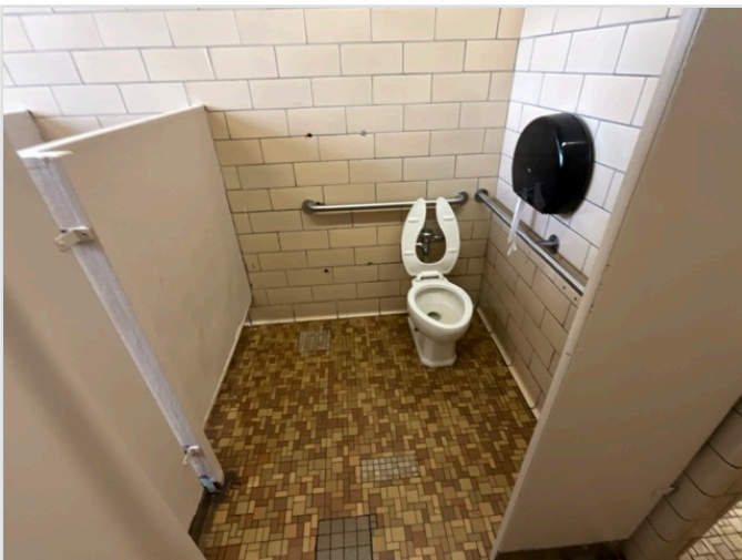
TOILET STALL OVERVIEW
