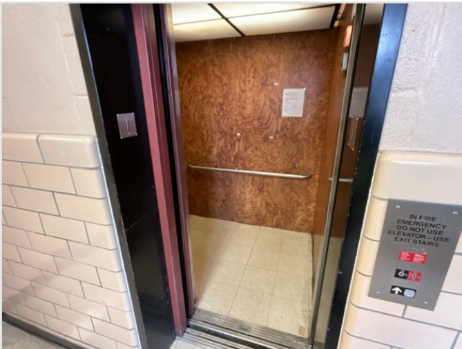
LOBBY LOOKING AT CABS
