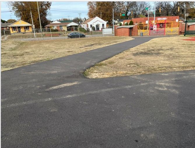
ACCESSIBLE ROUTE TO PLAYGROUND
