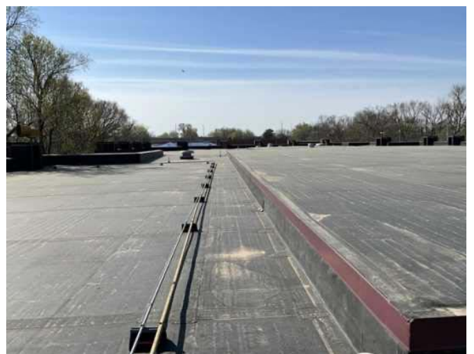
6 - EDPM ROOFING SYSTEM
