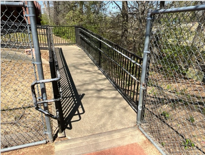
ACCESSIBLE ROUTE TO PLAYGROUND
