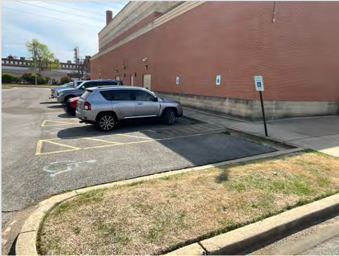
OVERVIEW OF ACCESSIBLE PARKING AREA
