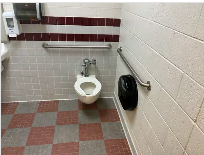
TOILET STALL OVERVIEW
