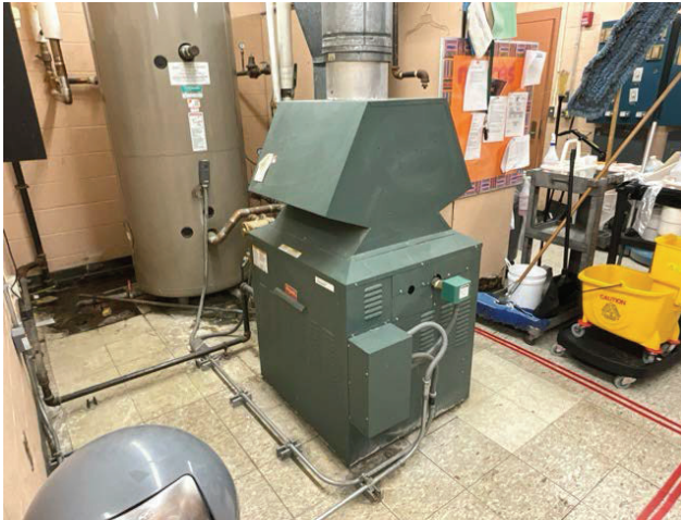
13 - DOMESTIC BOILER AND STORAGE TANK
