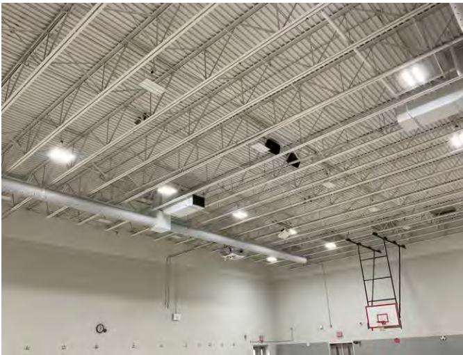
9 - GYM STRUCTURAL OVERVIEW
