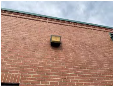
Many fixtures have damaged and yellow lenses. - AssetCALC ID: 7867463
