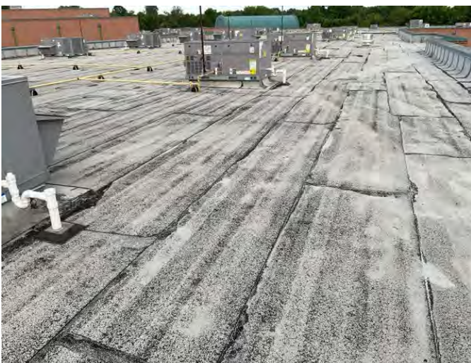
5 - MODIFIED BITUMINOUS ROOF
