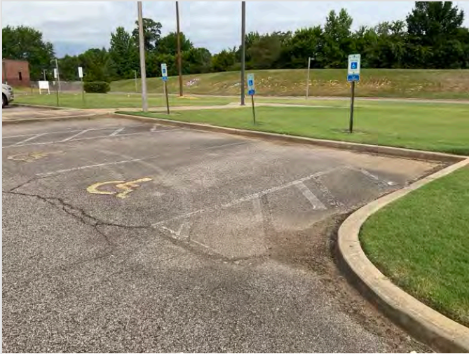
OVERVIEW OF ACCESSIBLE PARKING AREA
