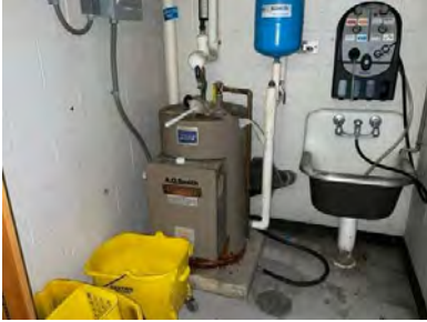
Leaking at base - AssetCALC ID: 7867547
