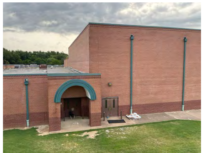
6 - BUILDING FACADE/ROOF DRAINAGE
