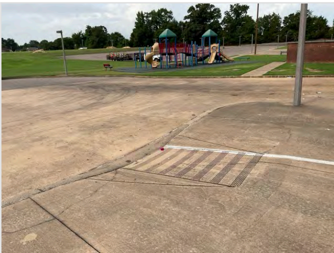
ACCESSIBLE ROUTE TO PLAYGROUND
