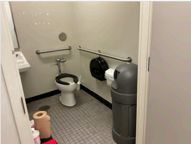
TOILET STALL OVERVIEW
