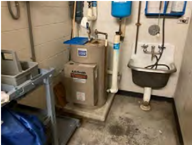
Substantial corrosion on top of water heater. - AssetCALC ID: 7867469
