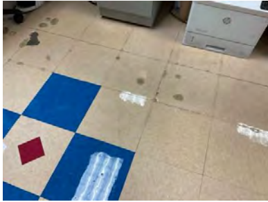
Damaged and stained VCT in office area - AssetCALC ID: 7867540
