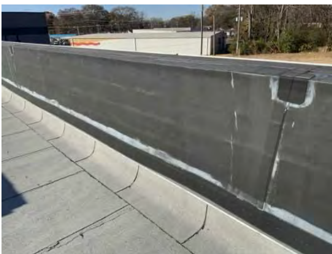
5 - EPDM ROOFING AT PARAPET
