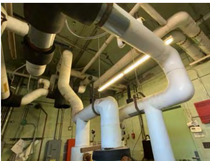
17 - DUAL TEMPERATURE PIPING
