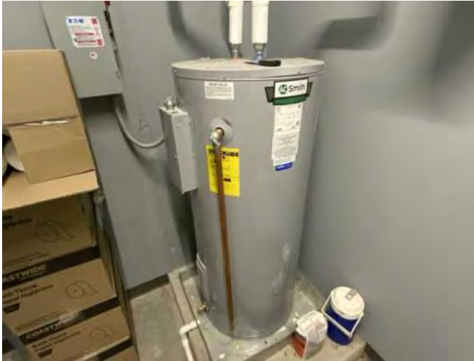
7 - ELECTRIC WATER HEATER
