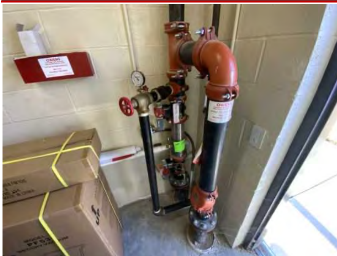
13 - FIRE SUPPRESSION CONTROL VALVE
