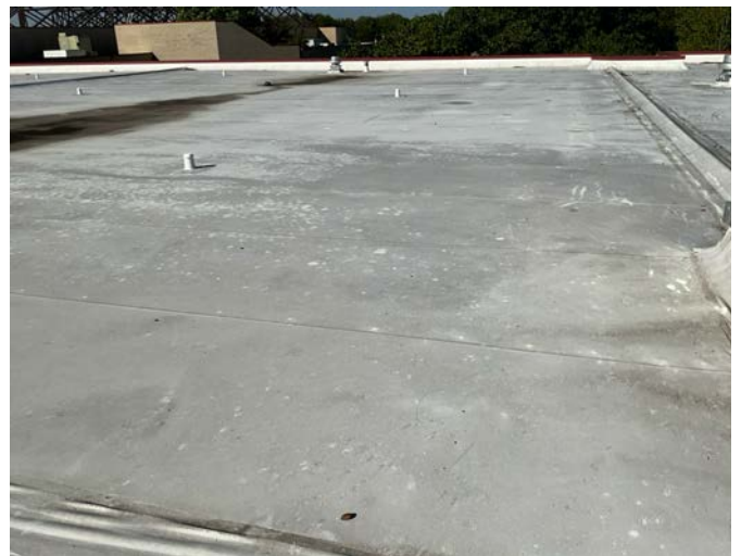
6 - ROOF NORTH VIEW
