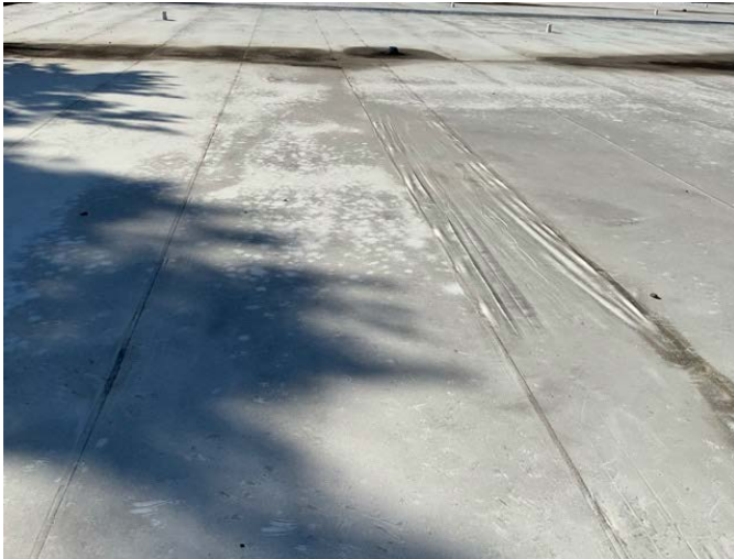
7 - ROOF SOUTH VIEW
