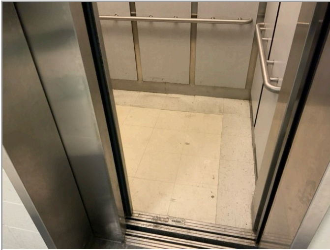
LOBBY LOOKING AT CABS (WITH DOORS OPEN)
