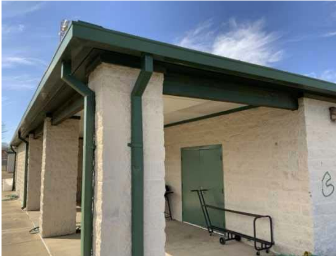
7 - CONCESSION RESTROOM BUILDING
