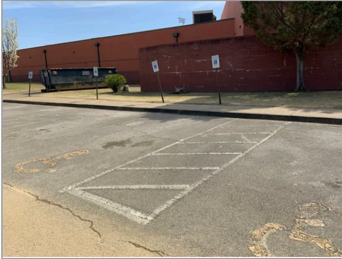
OVERVIEW OF ACCESSIBLE PARKING AREA
