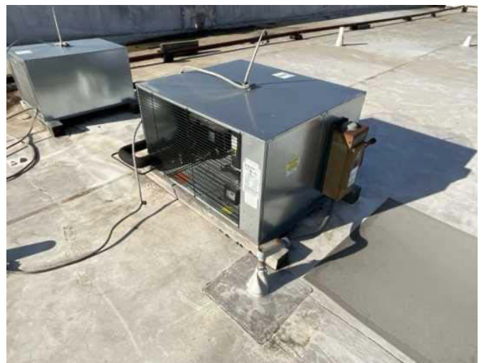
30 - REFRIGERATION COMPRESSORS
