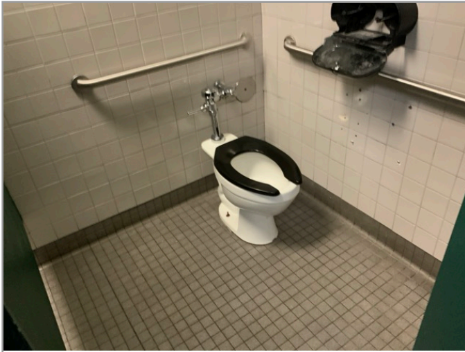
TOILET STALL OVERVIEW
