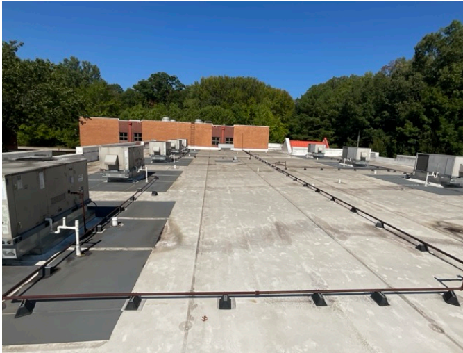
9 - PRIMARY ROOF OVERVIEW
