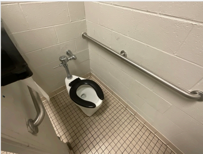
TOILET STALL OVERVIEW
