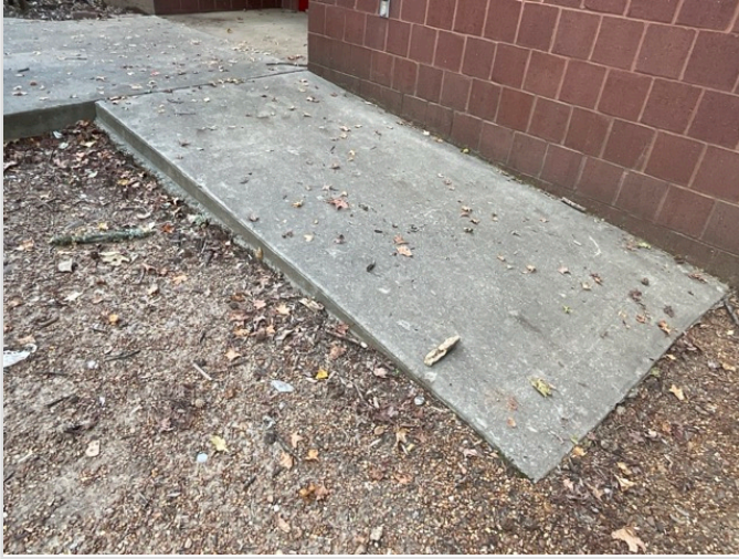
ACCESSIBLE ROUTE TO PLAYGROUND
