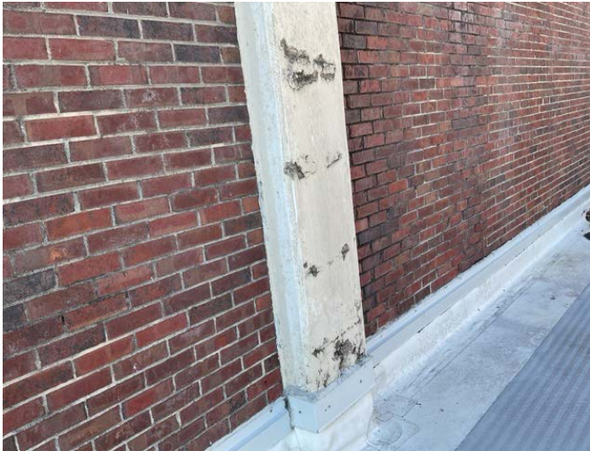
27 - SPALLED CONCRETE
