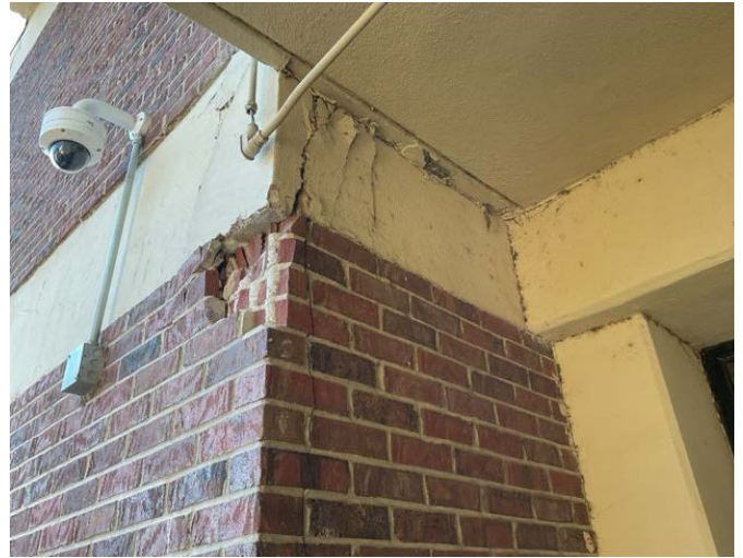
26 - EXTERIOR WALL DETERIORATION
