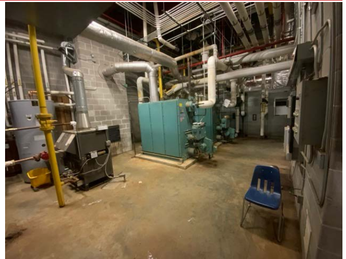
26 - MECHANICAL ROOM OVERVIEW
