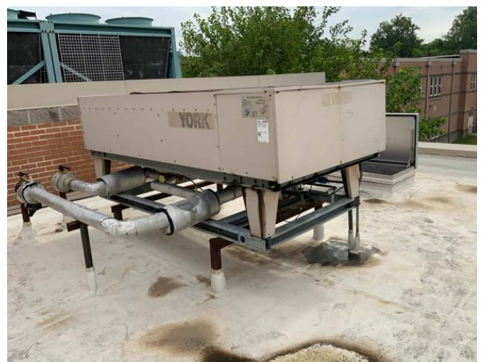
30 - SPLIT SYSTEM CONDENSING UNIT
