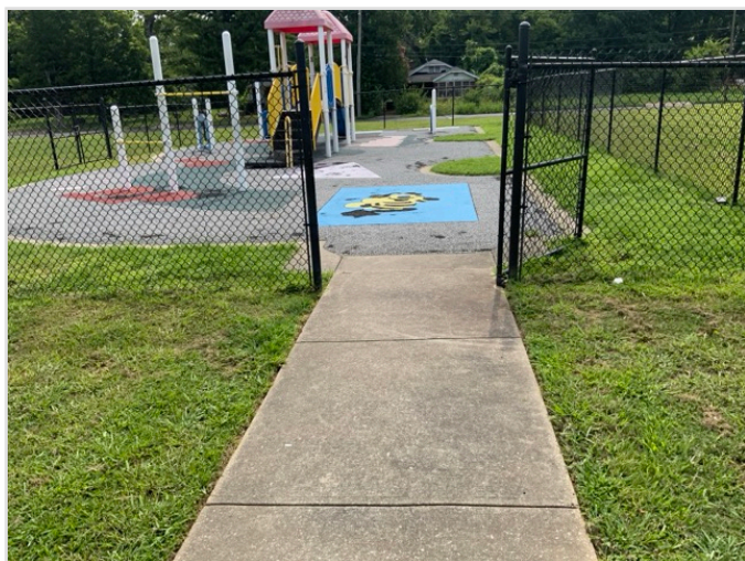
ACCESSIBLE ROUTE TO PLAYGROUND
