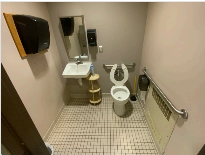
TOILET STALL OVERVIEW
