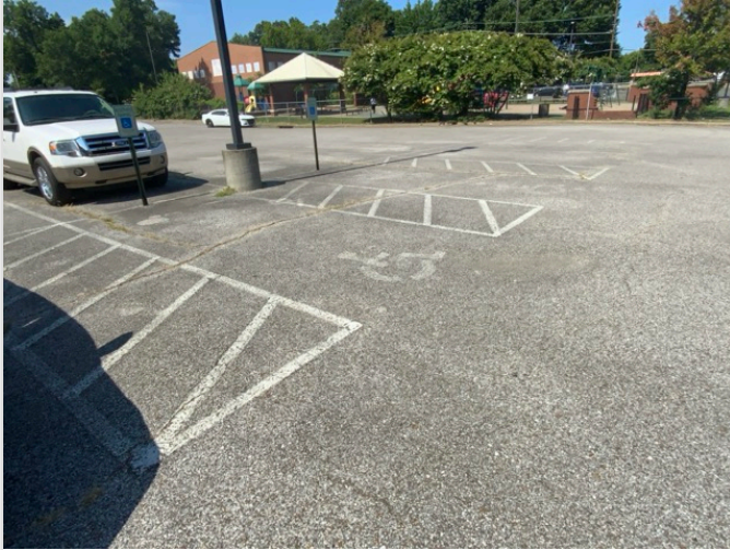
OVERVIEW OF ACCESSIBLE PARKING AREA
