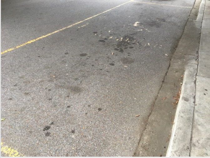
OVERVIEW OF ACCESSIBLE PARKING AREA
