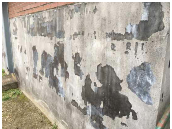
6 - EXTERIOR WALLS, CONCRETE, REPAIR
