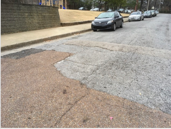
ACCESSIBLE ROUTE TO PLAYGROUND
