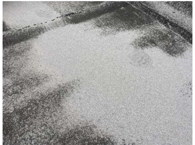
10 - ROOFING, MODIFIED BITUMEN
