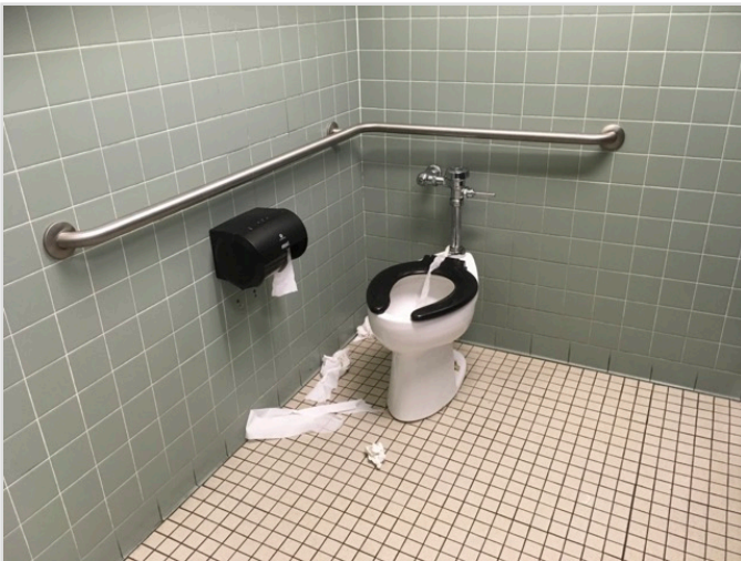
TOILET STALL OVERVIEW
