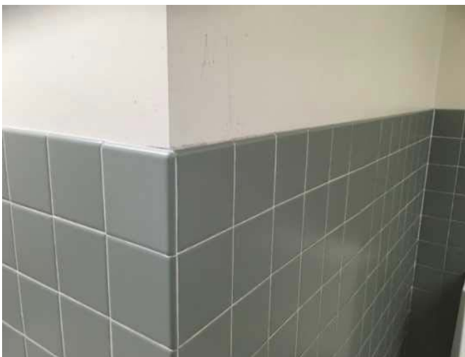
17 - WALL FINISHES, CERAMIC TILE
