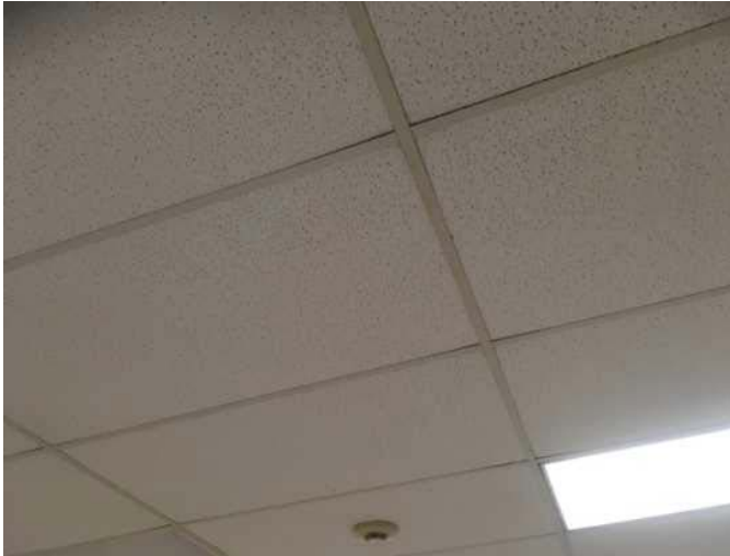
13 - SUSPENDED CEILINGS, ACOUSTICAL TILE
