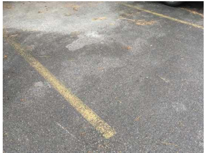
40 - PAVEMENT, ASPHALT, SEAL AND STRIPE
