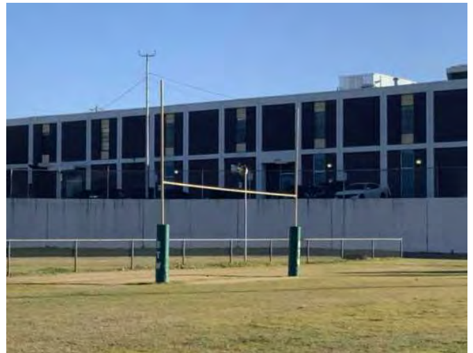
22 - GOAL POST AND RETAINING WALL
