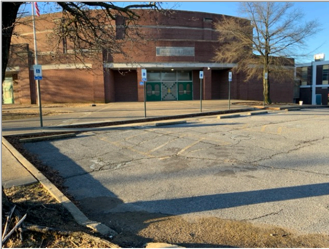
OVERVIEW OF ACCESSIBLE PARKING AREA
