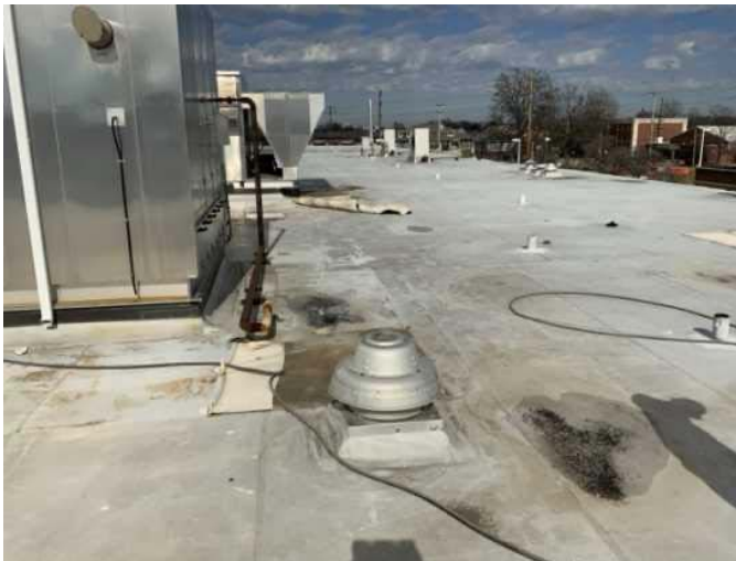
9 - PRIMARY ROOF OVERVIEW
