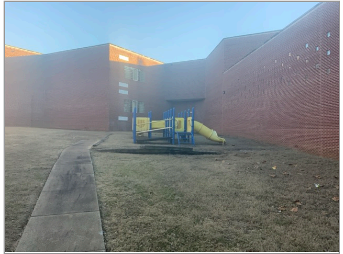
ACCESSIBLE ROUTE TO PLAYGROUND
