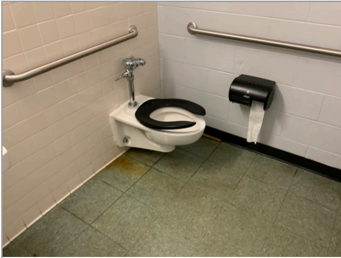
TOILET STALL OVERVIEW
