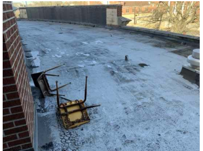
10 - SECONDARY ROOF OVERVIEW
