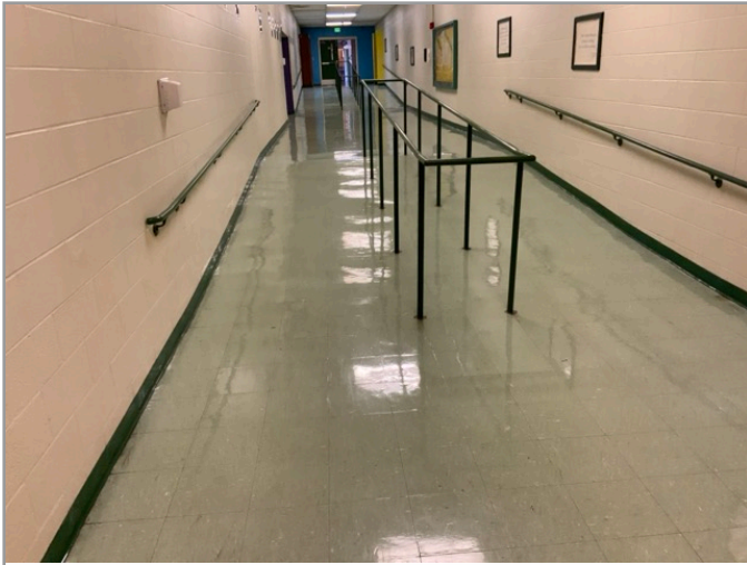
ACCESSIBLE INTERIOR RAMP
