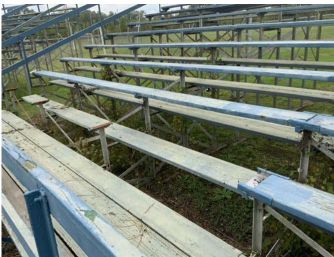
29 - BLEACHERS WITH MISSING BOARDS
