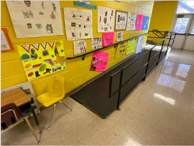
ACCESSIBLE INTERIOR RAMP
