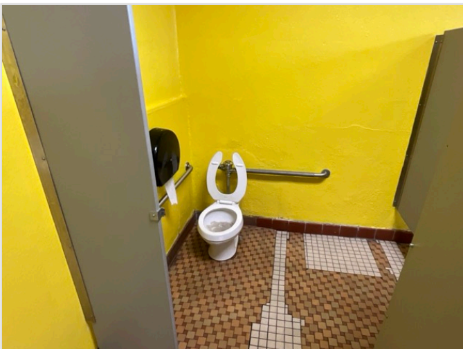
TOILET STALL OVERVIEW
