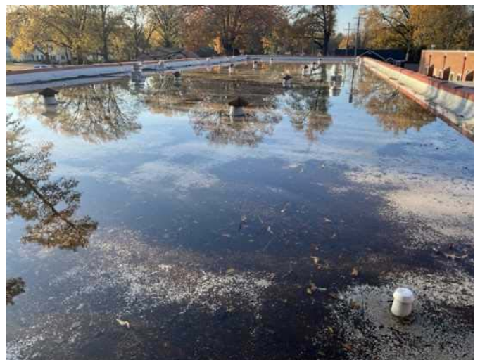
6 - ROOF DRAINS AND INTERIOR LEADERS
