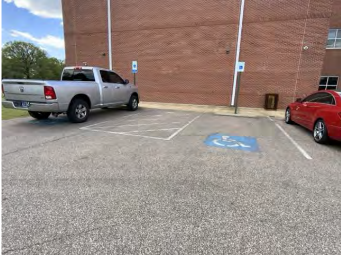
Overview of accessible parking area
