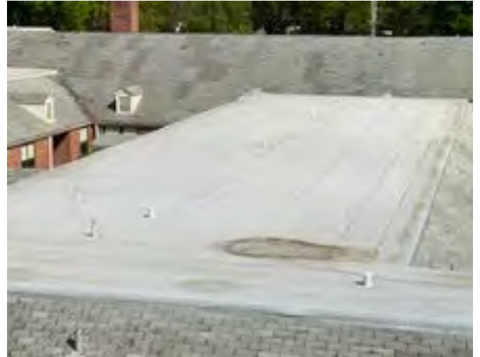
14 - MODIFIED BITUMEN ROOFING
