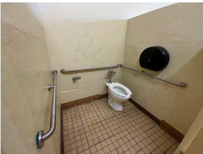
Toilet stall overview
