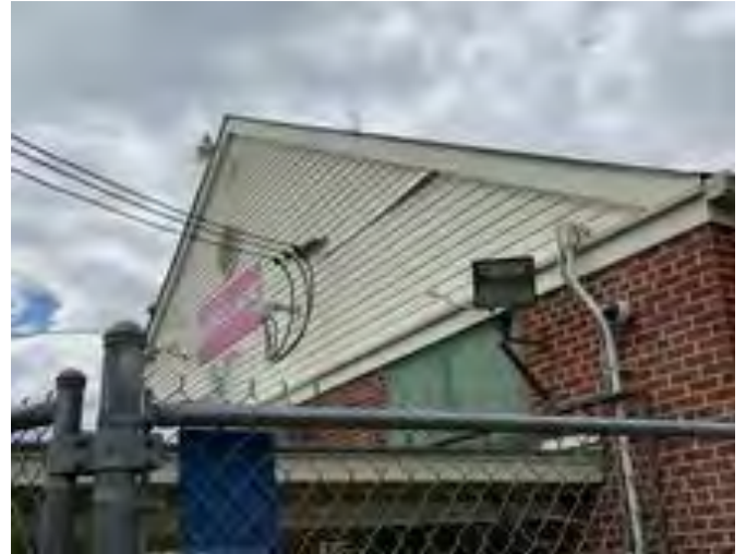
8 - EXTERIOR WALL SIDING
