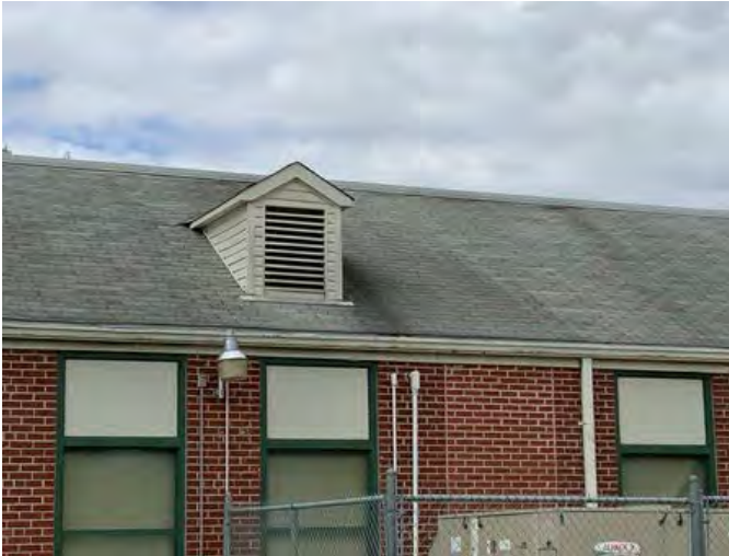
13 - ASPHALT SHINGLE ROOFING
