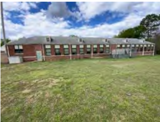
5 - OLD ANNEX BUILDING
