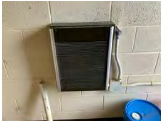
28 - ELECTRIC UNIT HEATER
