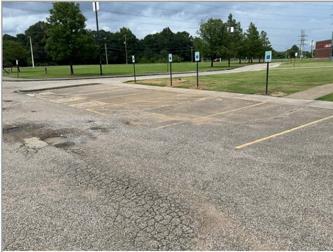
OVERVIEW OF ACCESSIBLE PARKING AREA
