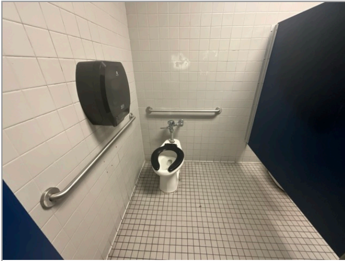
TOILET STALL OVERVIEW
