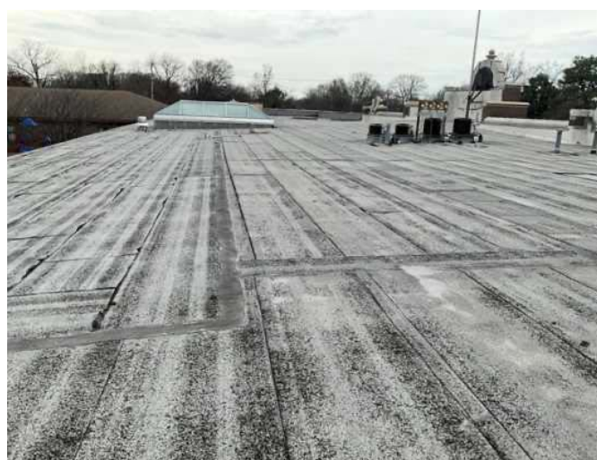
6 - MODIFIED BITUMEN ROOF
